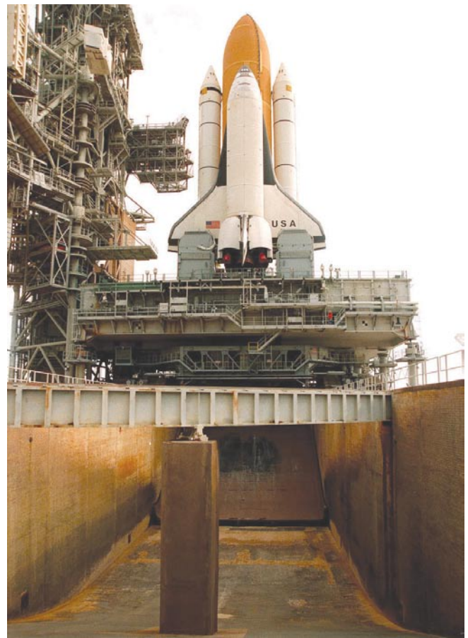
The Shuttle and MPLM sit above the flame trench.
