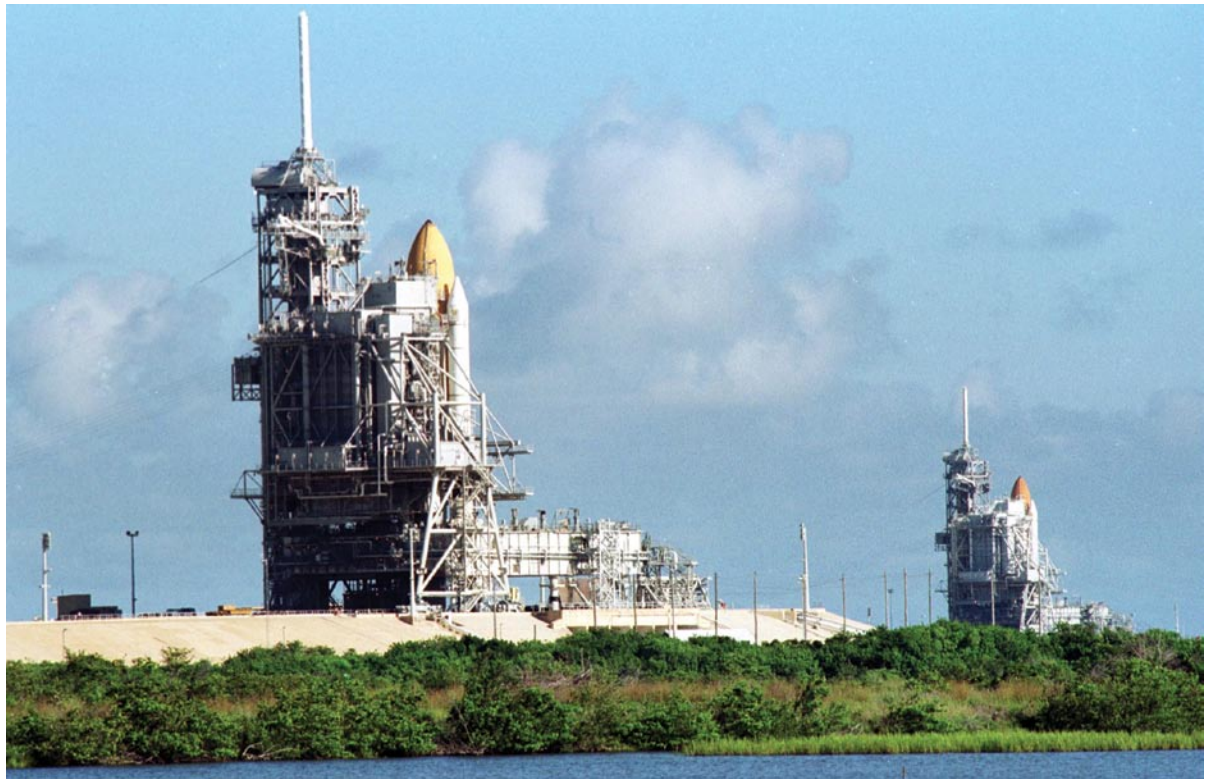
Space Shuttle Discovery (left) and Space Shuttle Atlantis (right) both stand ready on their Launch Pads (39A and 39B respectively). Atlantis launched first, July 12, 2001, on mission STS-104. Discovery launched Aug.10, 2001, on mission STS-105. Towering above each Shuttle at left is an 80-foot-tall lightning rod, part of the lightning protection system at the pads.
