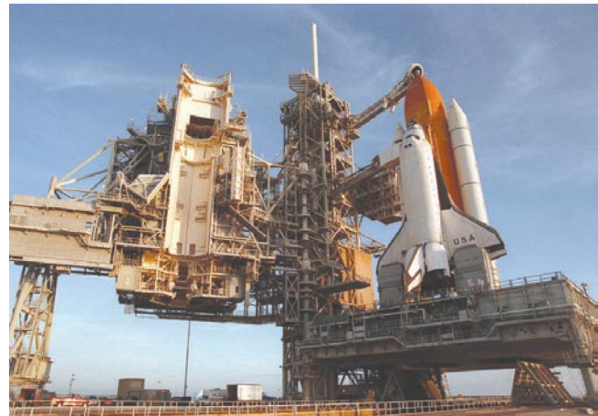
The Rotating Service Structure (left) is rolled open for launch. Entry to the Payload Changeout Room is exposed.
