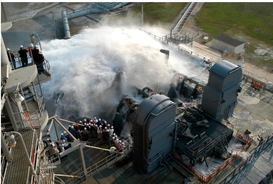
(Left) Water is released onto the Mobile Launcher Platform on Launch Pad 39A at the start of a water sound suppression test.
